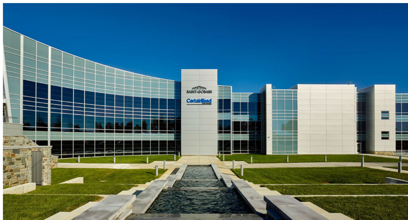
FACING PAGE The HQ boasts a cafe and fitness center, both of which were central to the entire design process and encourage employees to be healthy.
