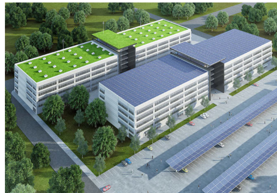
THIS SPREAD Pfister Energy provides engineering, procurement, and construction services for renewable energy projects.
