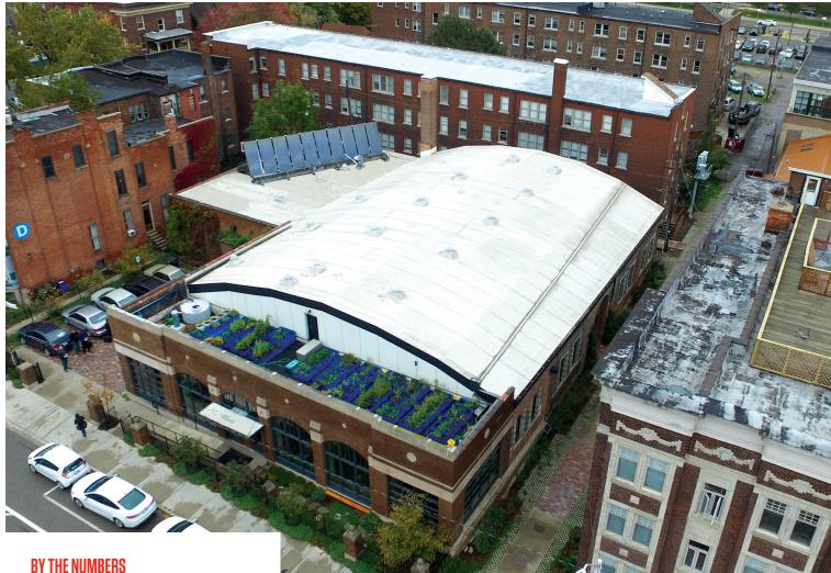
The Green Garage used solar thermal panels, not photovoltaics, as they were cheaper to install and allowed for a radiant loop heating system beneath the facility. Details:
