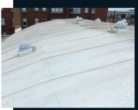
**GREEN GARAGE DETROIT** chose **DURO-LAST** for its roofing membrane because the product satisfied its primary objective-reduced heat absorption in warm months. It reflects up to 88 percent of the sun's energy, so the building interior requires less energy to be cooled. Additionally, pre-made rack flashings accommodated the thermal panels on the building annex roof, which heat the building in winter.
