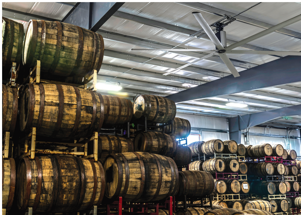
MacroAir installed large HVLS fans inside a Wisconsin brewery to keep patrons and workers comfortable and keep costs down.
