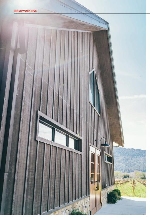
Venge Vineyards in California uses AWIP's customized wall panels and HR3 roof panels for a distressed wood appeal.
