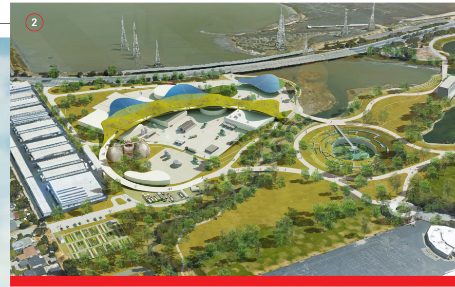
At the San Mateo Wastewater Treatment Plant, the design of the landscape provides storage for water at varying levels of flood conditions while maintaining pedestrian access through raised paths and bridges.
