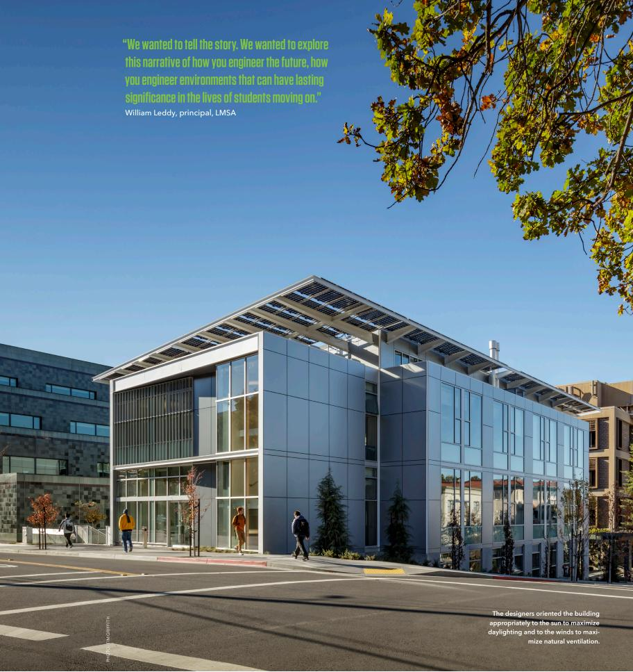
less energy and only adds appropriately supplemental cooling. Because the building opens to the prevailing winds, 100% of the instructional spaces above the basement level and 85% of regularly occupied spaces are naturally ventilated. When the windows are closed, mechanical ventilation provides 30% of added fresh air.
