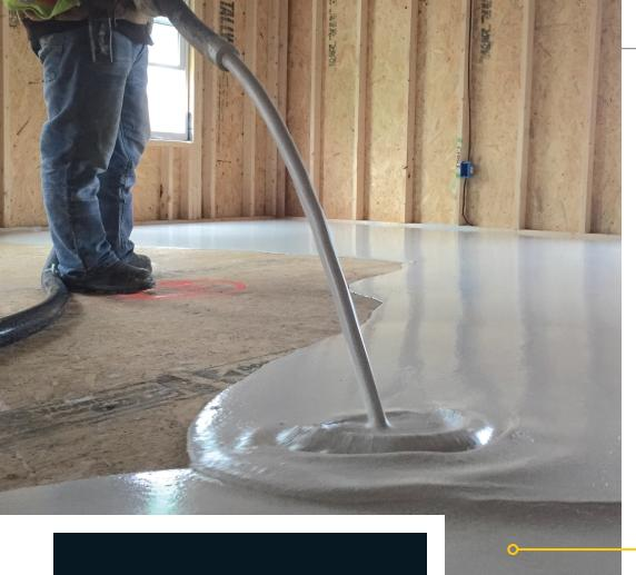
A small crew can pour up to 30,000 square feet of at three-quarters of an inch thick in one day, so it's less labor
